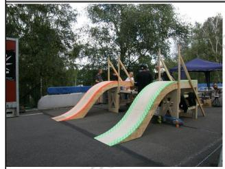
Ramps under construction are 125cm height, constructed in wood like the photo model with a s-shaped woody launch lane.
